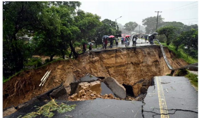
A road connecting the two cities of Blantyre and Lilongwe in Malawi has been torn apart by Cyclone Freddy. Photograph: Thoko Chikondi/AP
