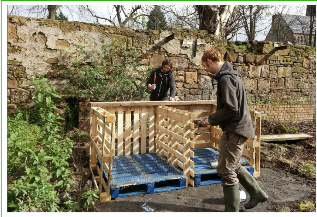
Pallet Bays at South Seeds
